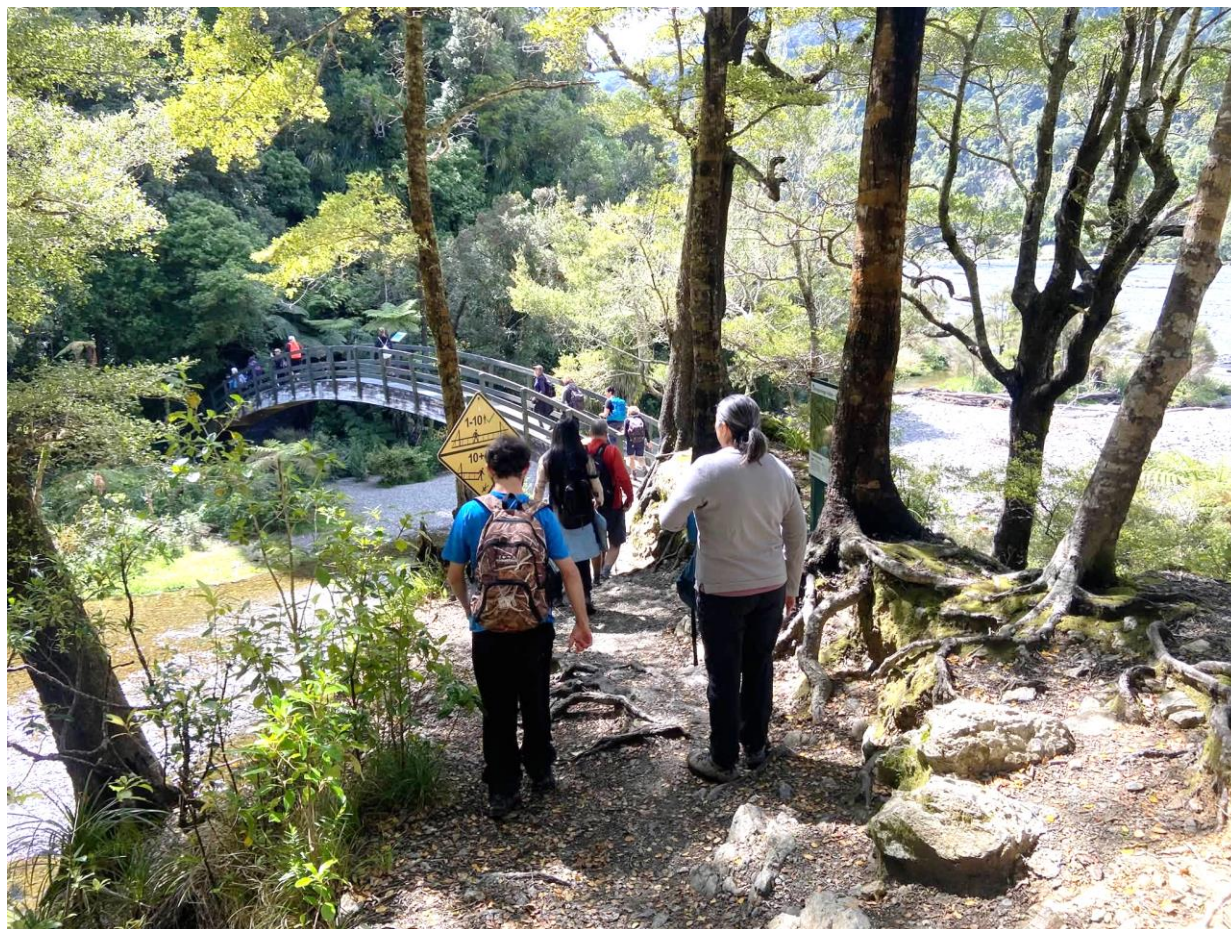
Turere Stream Bridge, 18 October 2026
